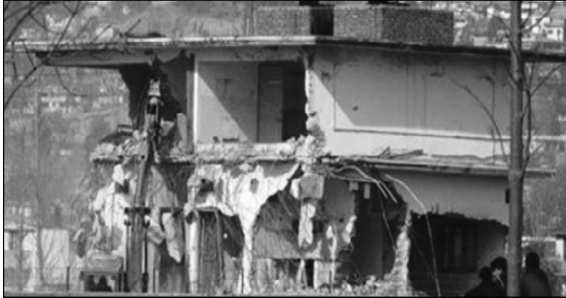
DEMOLITION ZONE: Cops stand guard as former al-Qaida supremo Osama bin Laden's safehouse in Abbottabad is demolished.
